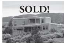
Eagle Ridge Road NE
